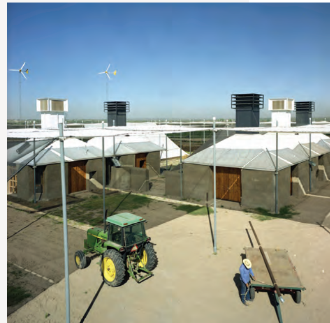
The Laredo Farm was designed on a grid using an economical, ecological, and regional material palette, which incorporated Buffel grass blocks supported by a wooden ladder block framing system, wrapped in chicken wire lath, and sprayed with fly ash-based cement. PHOTO BY R. GREG HURSLEY
