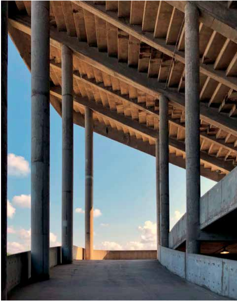
↑ Rice Football Stadium, located in Houston and designed by Lloyd and Morgan with Milton McGinty, 1950. The humble, symmetrical concrete stadium was profound when it was built.
