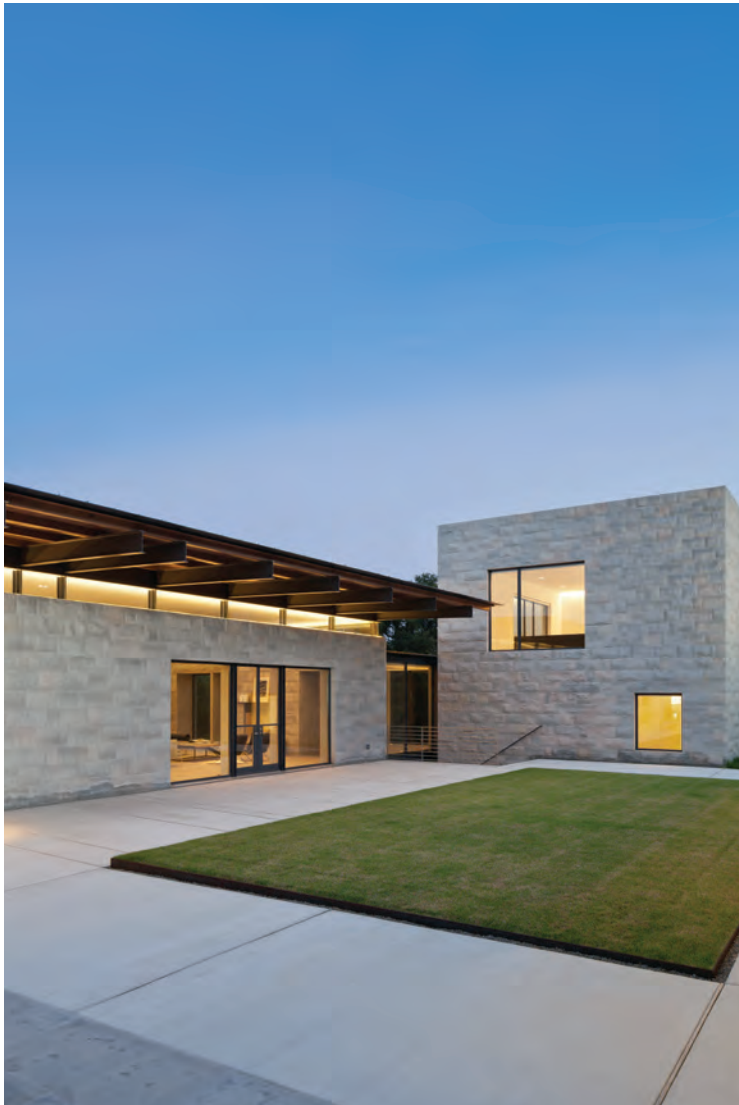
Lueders limestone, the dominant material used throughout the structure, is softened by patterning that refines the stone's heaviness. Clerestories accentuate the deliberate separation of elements.
