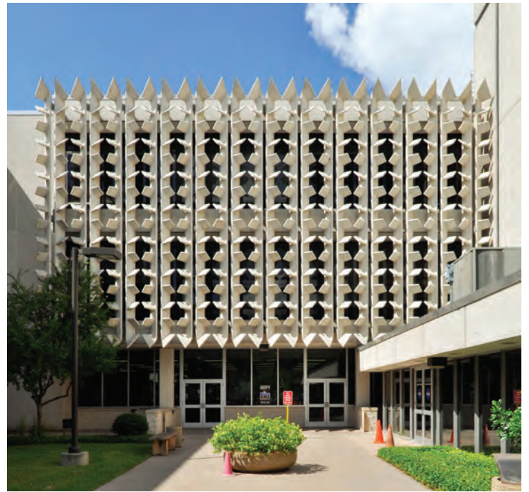
Right top and bottom The Johnson Space Center contains several nondescript administrative buildings that make extensive use of quickly assembled precast concrete panels. A concrete brise-soleil shades the entry lobby of Building 30.
