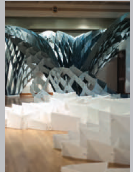
Left A full-scale prototype of 3xLP, built in collaboration with both Rigidized Metals and Zahner, demonstrates a range of possibilities for the project as a skin construct. Its rolled patterns and layered cross section are much more dynamic in terms of light diffusion and reflection than the team originally expected.
