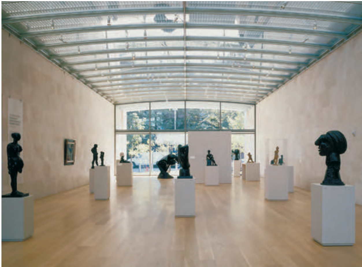
The Nasher Sculpture Center's roof, like that of the Menil, is a two-layer solution. In Dallas, the brise-soleil is positioned on the exterior of the glass, and recently, scrims have been added to the interior to mitigate the additional light reflected into the building.
