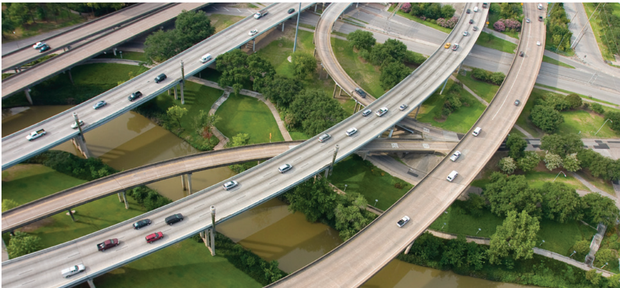
The Buffalo Bayou Promenade is woven through previously impenetrable highway interchanges. The project introduced 23 acres of parkland in Houston's inner city, linking downtown to the waterway.
