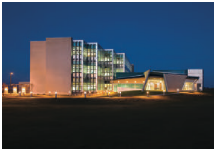
Richter Architects’ Harte Research Institute for the Gulf of Mexico Studies at Texas A&M University in Corpus Christi (top) and the National Museum of the Pacific War in Fredericksburg (bottom) both reference the history of the site and the significance of the program in their designs.
