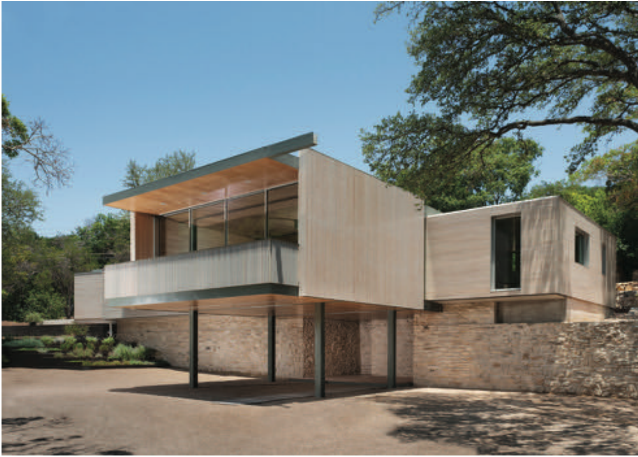
This page clockwise from top The new composition of crisp geometries sits above the rough stone wall retained from an earlier structure. The elevated living room looks out into the surrounding tree canopy. The crisply detailed construction is juxtaposed against rugged masonry.
