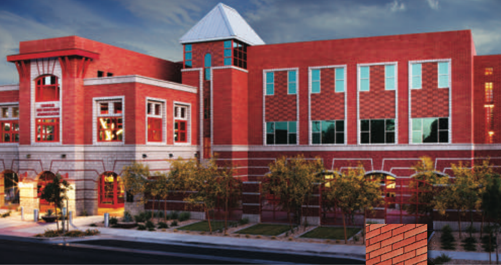
-Project: Chandler Fire Administration Building, Chandler, AZ.
