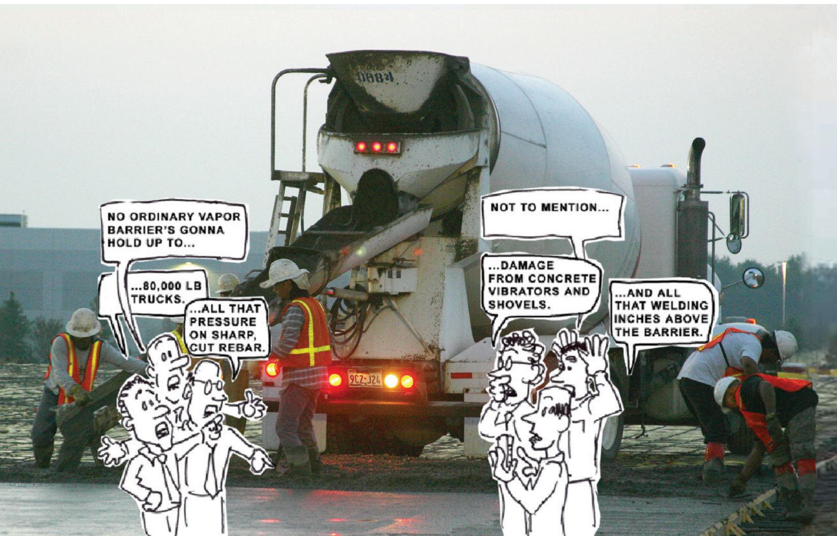
photo courtesy of constructionphotographs.com (File Name: concrete_pour_rebar_cement_truck_010.jpg) Graphics Modified
