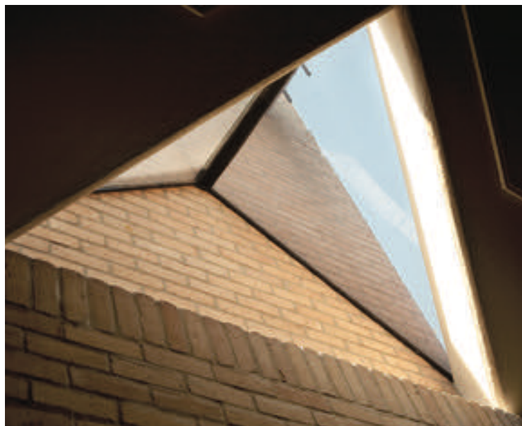
This spread, left to right David George with development sketches of a current residential project. Continuous open seam at roof ridge, Red Apple Inn. Gap between roof ridge and the chimney, George Residence.
