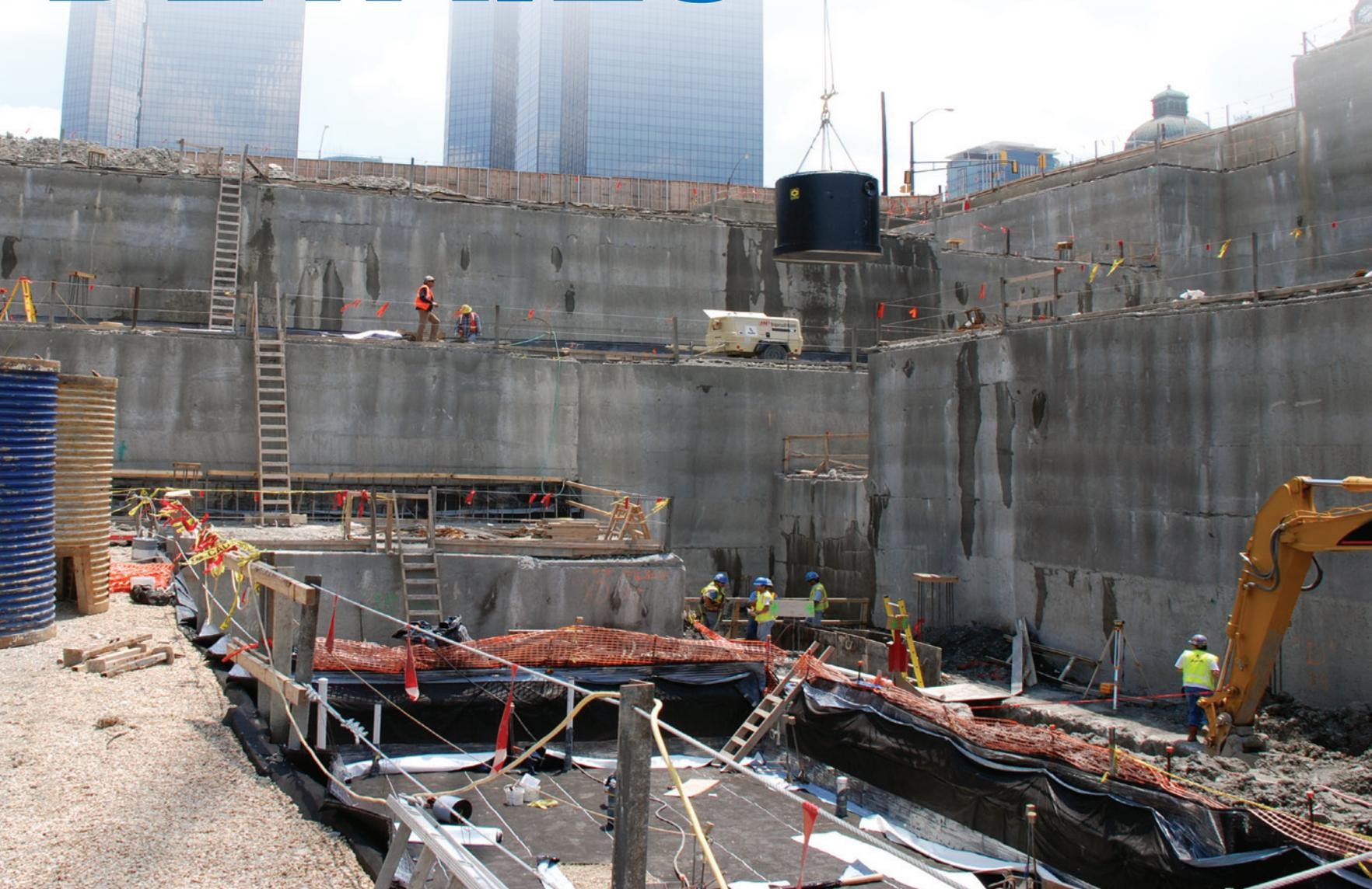
In building the Tarrant County College Trinity River East Campus in Fort Worth, Polyguard Underseal<sup>®</sup>, both Underslab and Blindsides, was used as waterproofing. As you can see, lots of detailing was required. Detailed areas are where most leaks occur throughout the building envelope.
