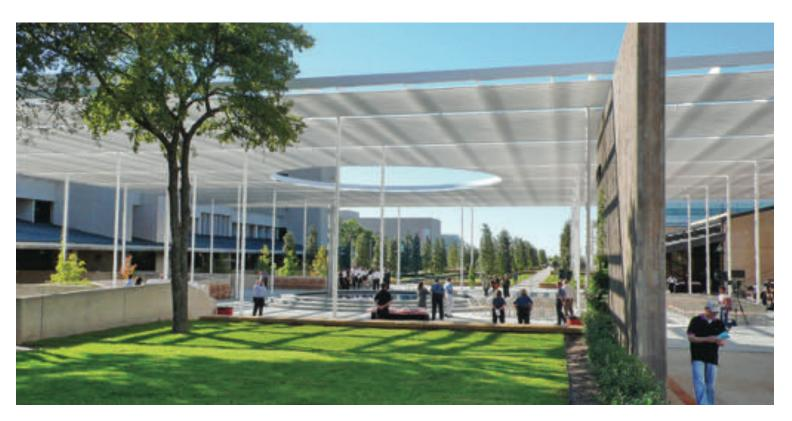
top and below The trellis, designed by Werner Sobek, is made from painted steel columns and beams that support fiberglass and plastic tubes. New construction will add 280,000 square feet to the campus by later this year.
