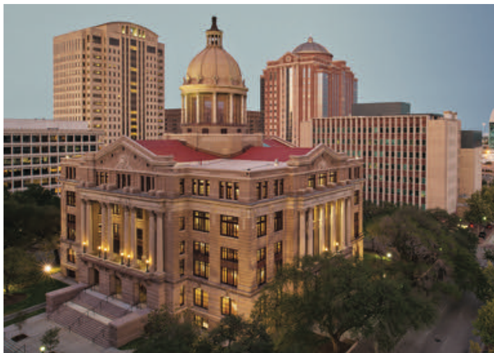
The Harris County Civil Courts Building, erected in 1910, originally served as the county's courthouse until its replacement opened in 1952. Following a $65 million restoration by PGAL, the six-story facility was rededicated on Aug. 23.
