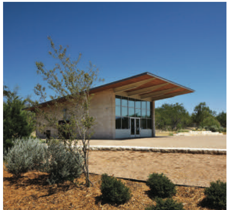
(opposite page, top and bottom) An oblique view shows the public egress at left, clerestory penetrations, and the entry's dramatic overhang. The curved pedestrian path winds through the entire building.
