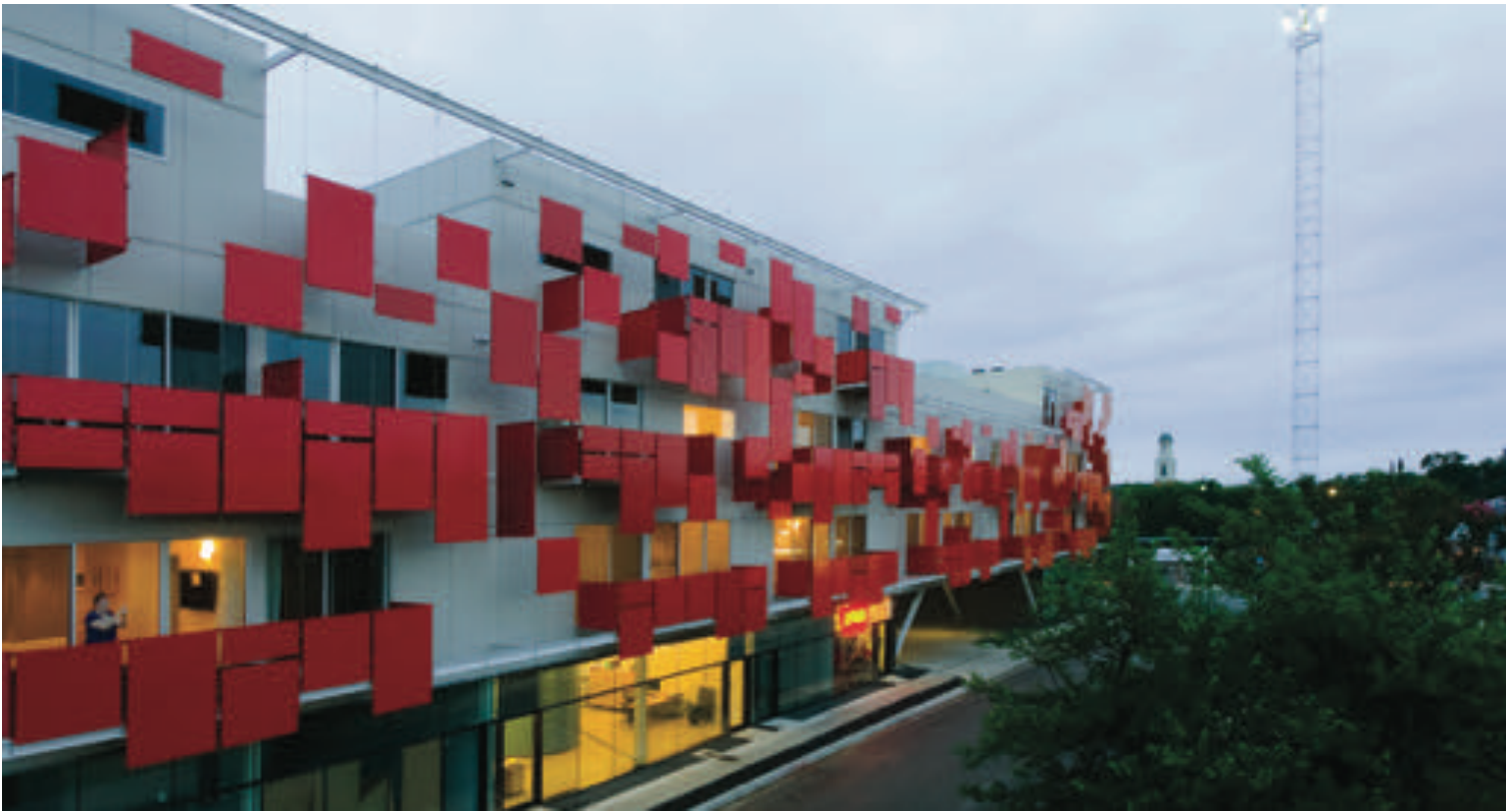
(above) The architects notched two terraces into the fourth-floor level, which will be planted with vegetation and accessible to all as a tenant amenity.
