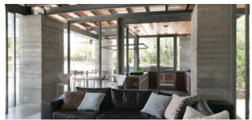
each plank in the formwork to produce deeply extruded horizontal ribs in random patterns across each face. This technique emphasizes textural changes in direct sunlight, and varying shadows define and amplify the richness of the concrete masses throughout the day.
