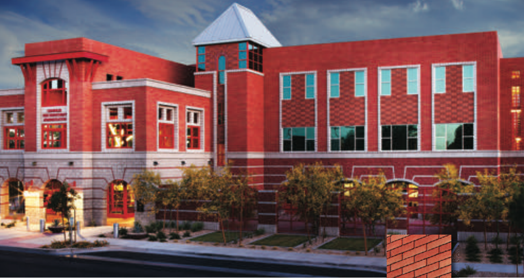
-Project: Chandler Fire Administration Building, Chandler, AZ.
