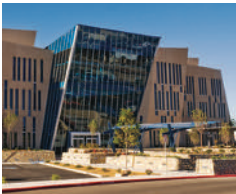
GECU Central Operations
