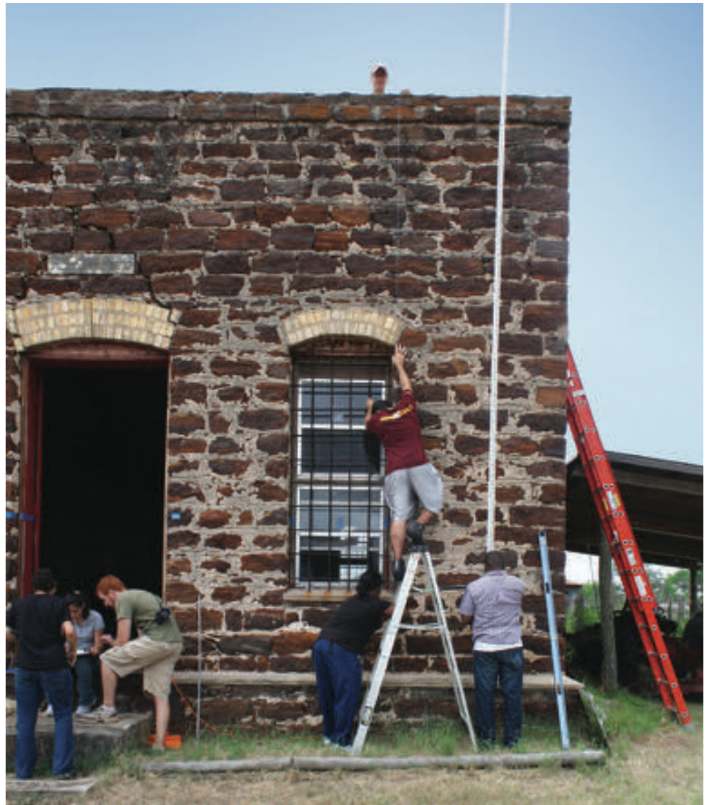
UTSA students took measurements of the Heermann Store prior to producing a set drawings based on the standards of the Historic American Building Survey. The one-room structure of load-bearing, rough-cut, coursed blocks of red sandstone dates from 1892 and was erected along the Rockport Road (now re-aligned to form Loop 1604 in southwest Bexar County), which connected Castroville and the Texas coast.
