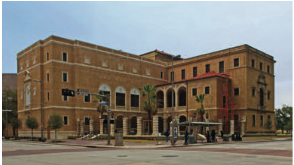
The recent expansion of the historic Julia Ideson Building in downtown Houston added a new 21,500-sf wing, shown at left, and an enclosed garden in front. An interior restoration of the original 1926 building will continue through next spring.
