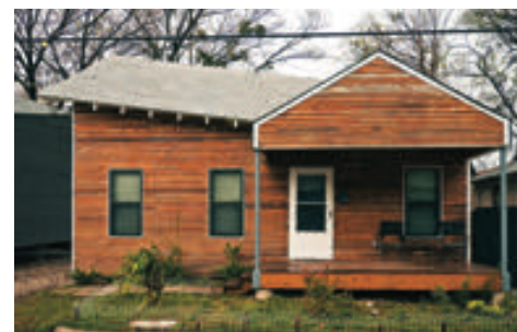
Congo Street House—After
