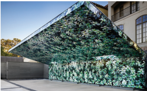
Meredith Long Gallery Carport and Parking Plaza
