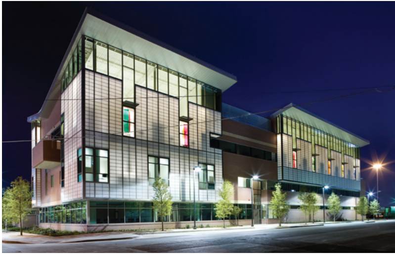
(top) The dining pavilion opens to the central courtyard with an entry protected by a high canopy.
