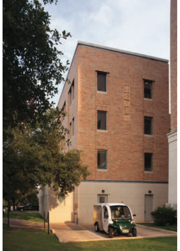
(preceding spread, clockwise from far left) Cooling towers crown the new Chilling Station No. 6, built on a tight site on the east side of the UT Austin campus. Adjacent to the chiller facility is the expansion of the Hal C. Weaver Power Plant. The north facade of the expansion project complements the ACES building next door to the west. (above) Relief panels set in the new Weaver building's northwest corner denote its industrial function.
