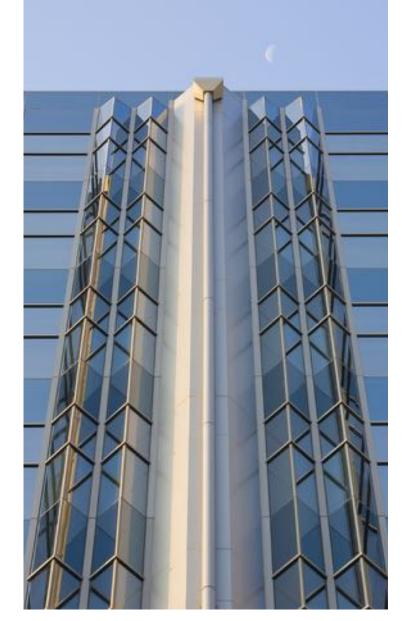
(preceding spread) The Margaret M. Alkek Building for Biomedical Research was completed in 2007. (this page, top) Lord Aeck & Sargent's architecturally expressed roof drainage system is integrated into metal columns. (this page, bottom) The metal armature casework systems provide visual lightness and functional flexibility to lab arrangements.
