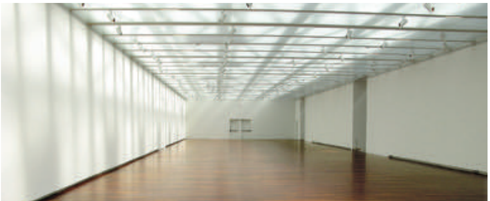
The design team devised a unique roof system to protect artwork from the South Texas sun, with fixed metal louvers at the top and moveable panes of fritted glass at the ceiling level that electronically adjust to light conditions.
