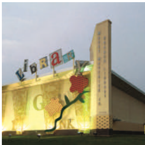
Fire Station No. 49/Maury Maverick Jr. Branch Library
