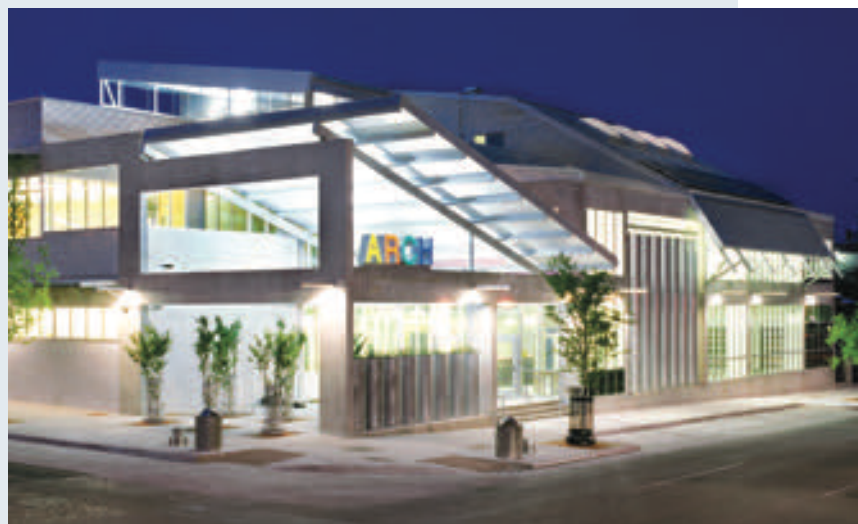
The Austin Research Center for the Homeless (ARCH) designed by LZT Architects uses a site-poured, stacked concrete frame. To meet the standards of LEED Silver Certification, designers mixed a high volume of flyash into the concrete.
