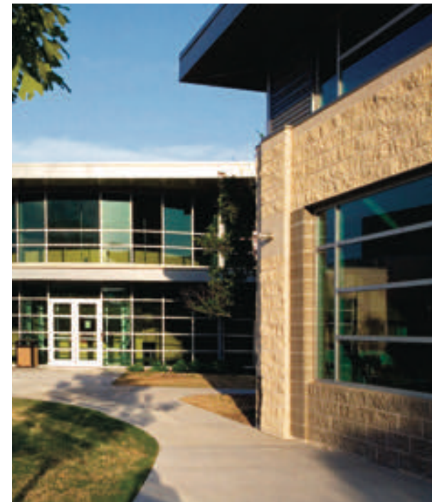
(top left) The V-shaped lower school includes a central, open area for learning activities. (top right) At the center of the middle school is the Beit Kneset, an interior gathering space for study and worship. (here and at right) Materials were selected for scale and durability.
