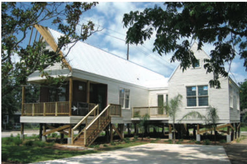
MC2’s design for the Ngyuen residence (top) incorporates a mid-level porch to connect the family with the outdoors, particularly a large oak in the back yard. Brett Zamore Design altered its original concept for the Parker residence (bottom) by turning a courtyard stair to open toward the street.
