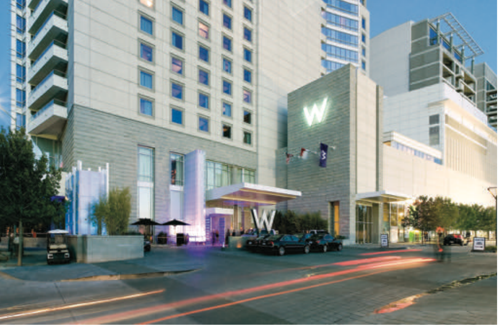
(above) Textured Lueders limestone grounds the base of the building. (opposite page) Early drawings illustrate the varied profiles of the 33-story tower.
