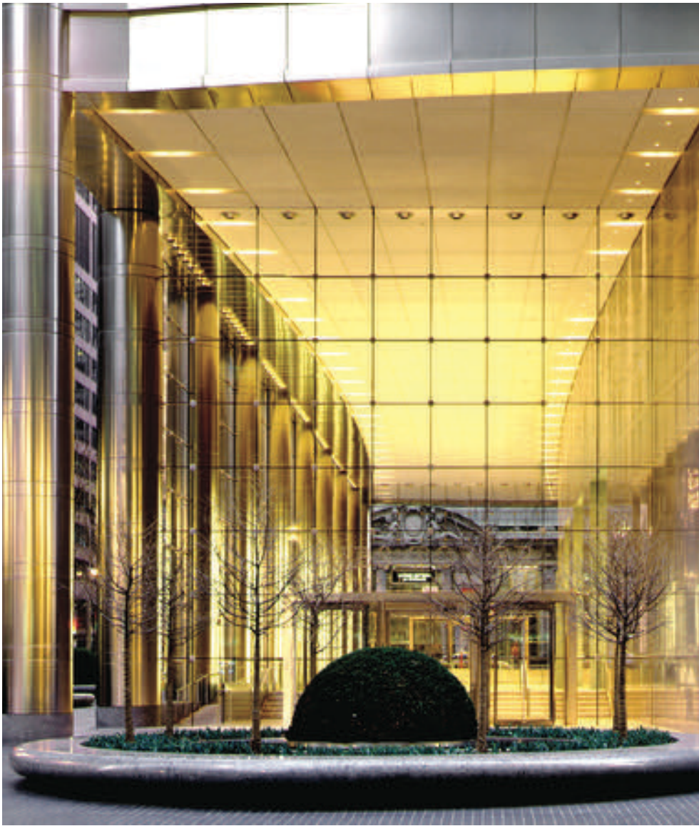
The lobby of One North Wacker in Chicago has a cable net glazing system with low-iron, anti-reflective glass. The architect is Goettsch Partners, formerly Lohan Caprile Goettsch, of Chicago.
