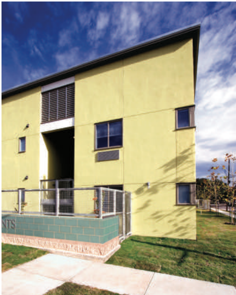
(top left) The residential component of the building, shown at the southeast corner, features a small fenced area of yard that runs along busy Canal Street. (top right) A typical 210-sf apartment within the 133-unit complex.
