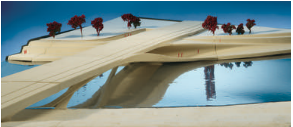
The North Main Street Bridge, planned to span the river between the 800 and 900 blocks, is designed to be 351 feet long and 72 feet wide. Three curvilinear arches will support four lanes of roadway.
