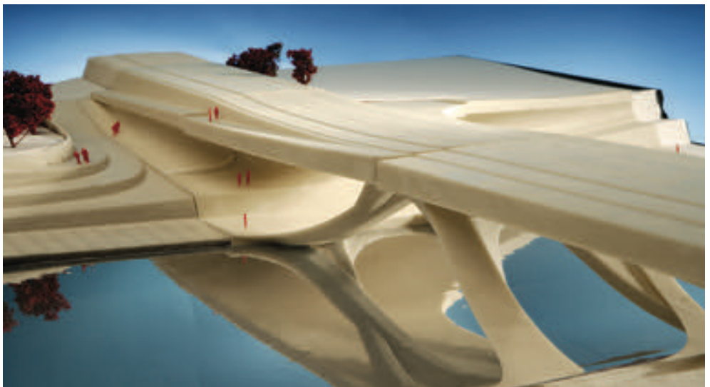
White Settlement Road Bridge, located between the 2000 and 2400 blocks, is designed to be 317 feet long and 72 feet wide with four lanes. Four arches will cross the underside of the span.
