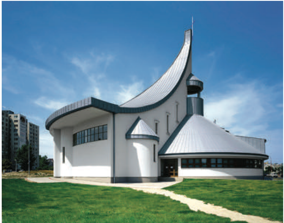
The Church of the Holy Spirit in Bratislava, Slovakia, uses preweathered titanium zinc in a blue-gray tone. The material, altered to resemble naturally aged zinc, forms the 14,961-square-foot roof and the facade's angled standing-seam panels.
