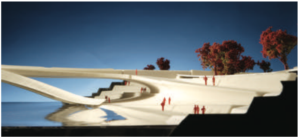
Henderson Street Bridge will stretch 367 feet between the 800 and 900 blocks. At 100 feet wide, the span will incorporate five sweeping arches to support four lanes that may be extended to six.
