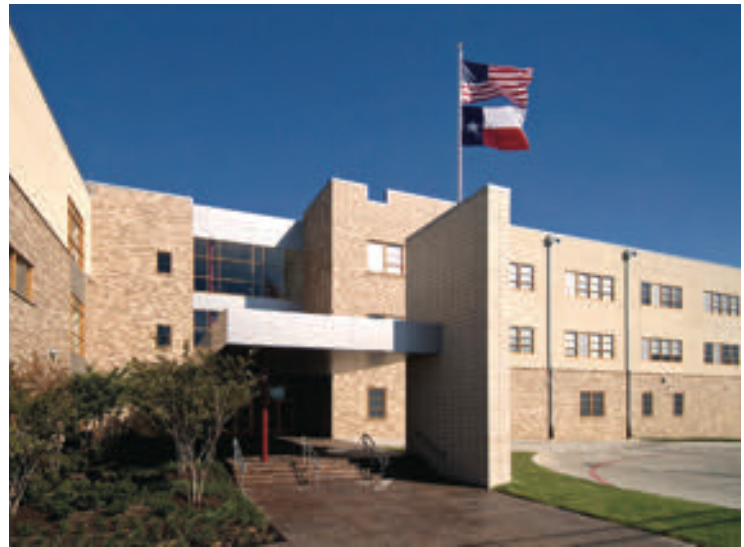
Challenged by scarcity of land in a densely populated neighborhood, BRW Architects combined Tasby Middle School (above) and Lowe Elementary onto a single site.
