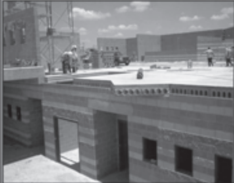
New Elementary School at LaGrulla ISD
