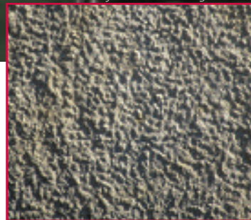
A brush-hammered finish created an aged texture.
