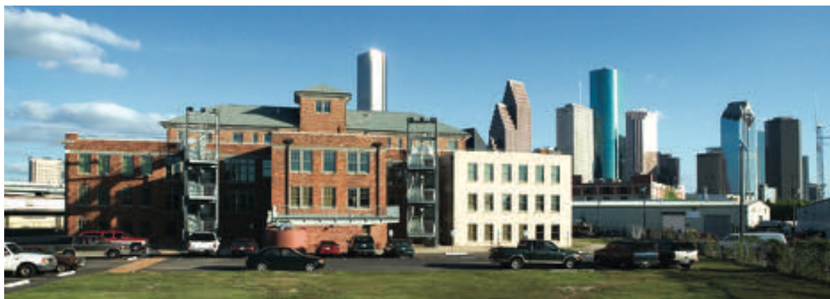
The rehabilitated Jefferson Davis Hospital is now the Elder Street Artists Lofts, with a planted roof on the three-story addition at the far right.
