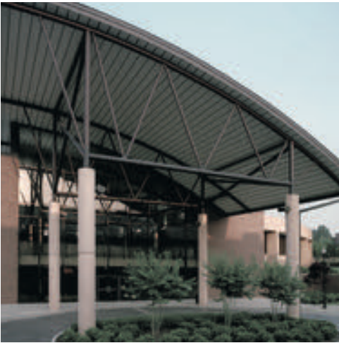
TWH ARCHITECTS, INC., TENNESSEE
