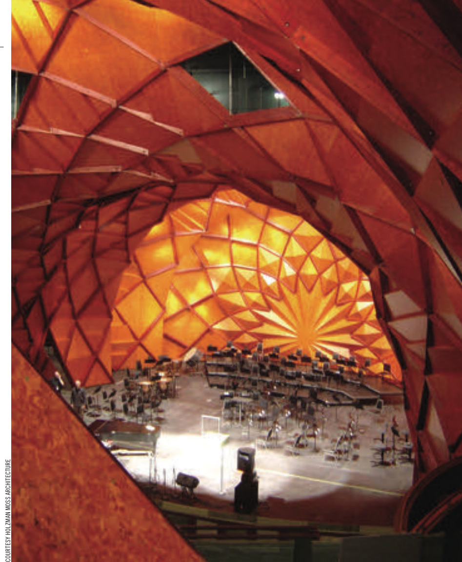
At the recently completed Globe-News Center for the Performing Arts in Amarillo, Holzman Moss Architecture devised a movable orchestra shell constructed of glulam timber and oriented strand board panels. Each panel was specifically designed to correctly reflect sound waves from the stage.
