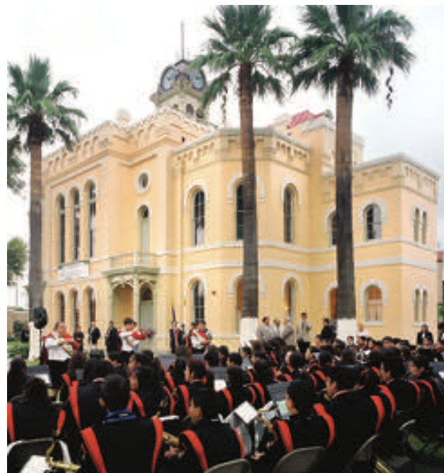
The Maverick County Courthouse, designed by Wahrenberger & Beckman and built in 1885, was rededicated in October 2002. The San Antonio firm Ford, Powell & Carson led the $2.9 million restoration project.
