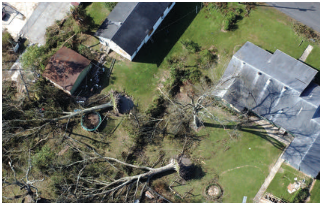
Orange County was among the regions in Texas most damaged by Hurricane Rita after she made landfall off the Gulf coast early on the morning of Sept. 24.
