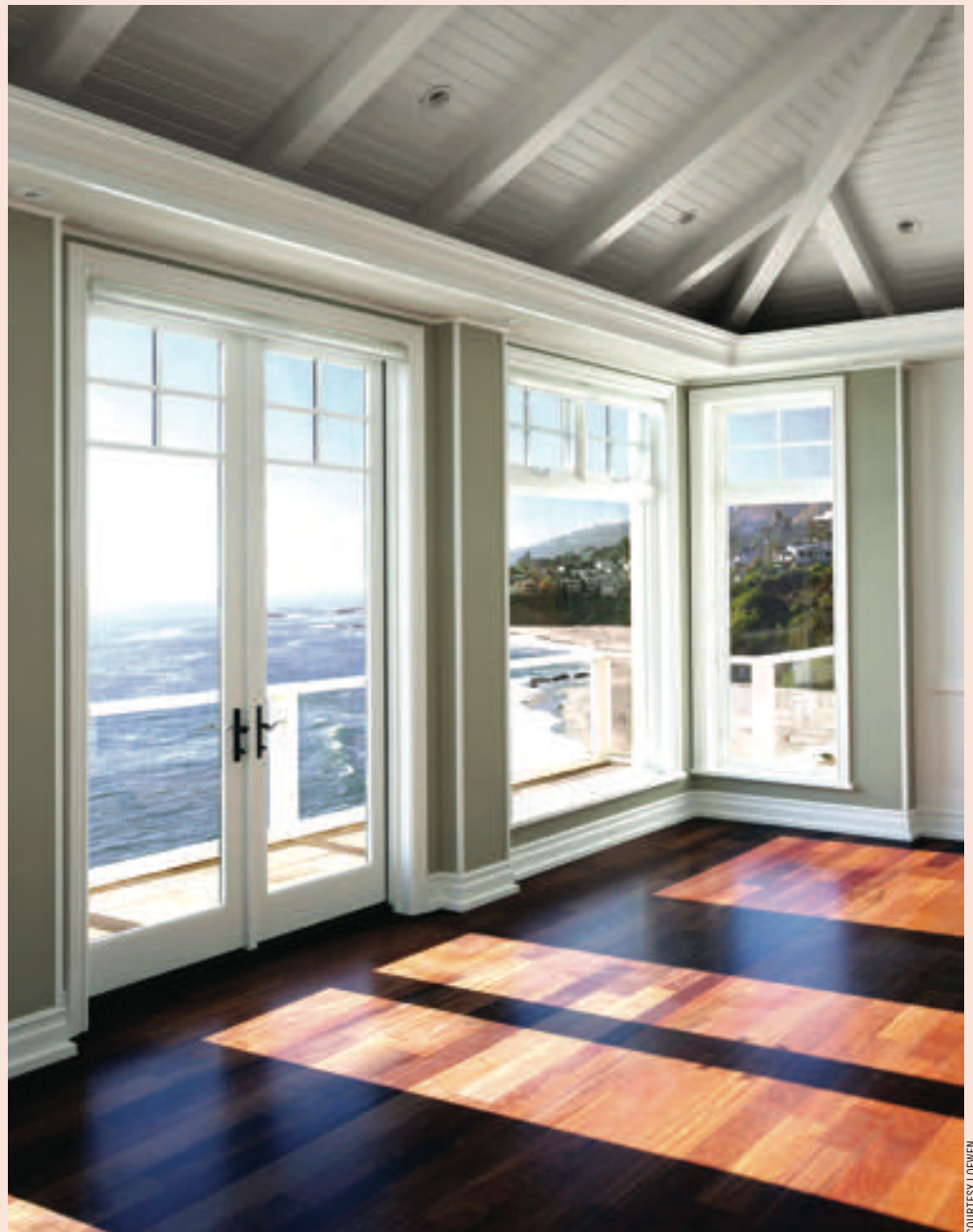
Hardwood flooring is a popular choice for residential and commercial building types. The residential project illustrated above uses mahogany hardwood, which is ideal for domestic applications because of its hardness and color fastness.
