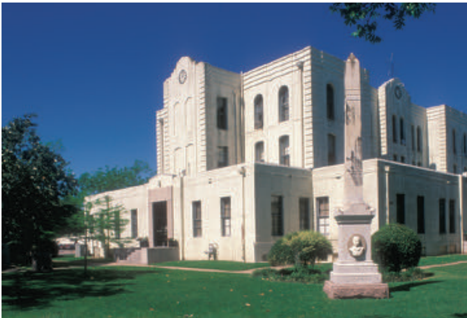
Extensive remodeling in the mid-1900s, including the removal of the courthouse tower, completely transformed its facade in an attempt to modernize the structure.
