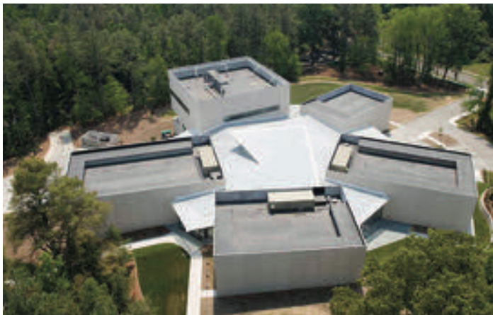
Roof-top clerestory introduces daylight into the three gallery spaces.
