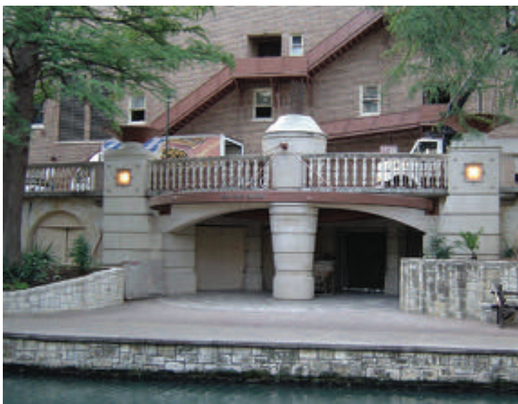
Overland Partners' Aztec Theatre Riverwalk Improvements in progress in October.
