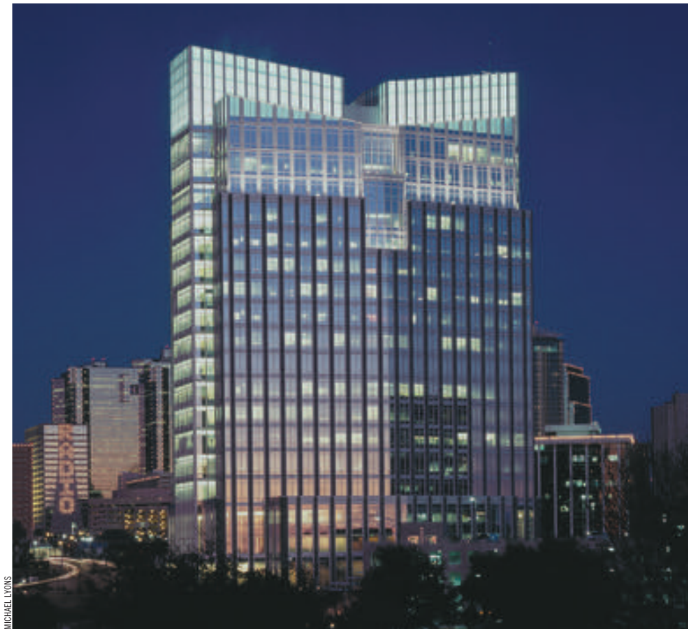
While some types of HID (high-intensity discharge) lamps are not recommended for critical lighting applications, they are commonly used for outdoor and large area applications. For example, metal halide spot and flood fixtures add to the dramatic presence of Duda/Paine Architects' Pier 1 Place on the Fort Worth skyline.
