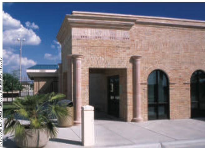
Starr-Camargo Port of Entry's projecting cornice, decorative frieze, and Doric columns reflect Portscheller's 1886 Río Grande City masterpiece.
