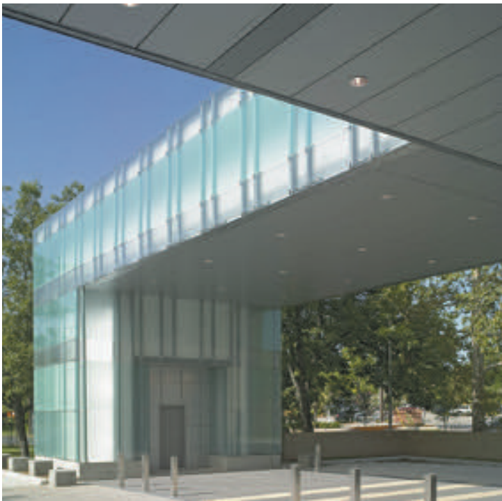
Seton Medical Center Expansion and Renovation by Page Southerland Page
