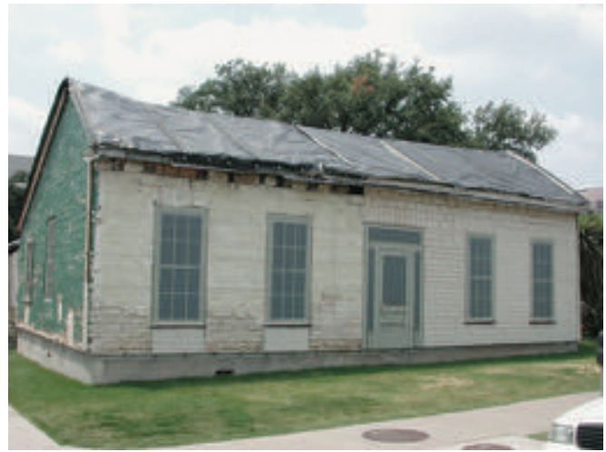
Relocated to a downtown Austin public park, the circa-1870 home of Susanna Dickinson awaits further funds for preservation. Volunteers have painted a faux facade on the house to approximate the structure's original detailing; photo by Wayne Bell, FAIA
