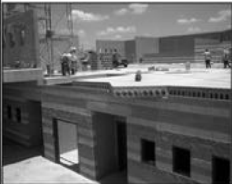
New Elementary School at LaGrulla ISD
