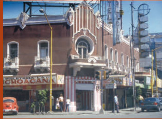
Colegio Cervantes reinterprets the rich, neoclassical tradition of late nineteenth- and early twentieth-century brick and masonry architecture of Torreón. These structures typically feature, among other qualities, elaborate cornice details which created modulated shadows in the bright light and desert heat. This tradition evolved during the 1930s to include eclectic, Art Deco-inspired work such as the Hotel Galicia (shown here) on Torreón’s downtown plaza.
