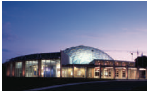
Casa Mañana Theatre Renovation and Expansion
