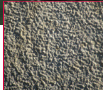
A brush-hammered finish created an aged texture.
