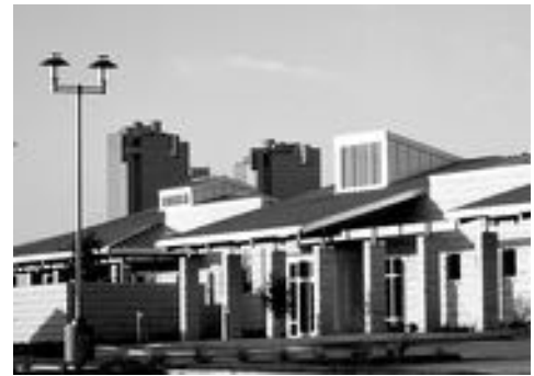
Tarrant Regional Water District Administration Building
