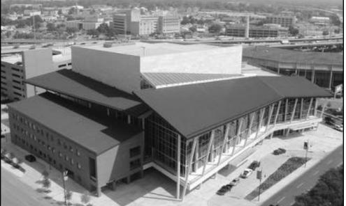
Berridge's Cee-Lock Standing Seam Roof System provides the distinctive finish to the angular, skewed roof shapes of the new Hobby Center for the Performing Arts in Houston. Berridge "Colonial Red" Kymar 500<sup>o</sup> finish contrasts dramatically with limestone. class, and brick walls. and steel columns. as well as the urban surroundinas.
