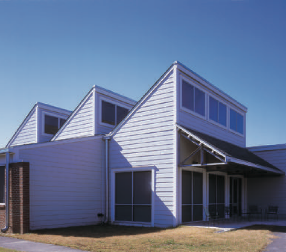
(top) The jagged roofline and choice of materials differentiates the cottages from the older buildings and create a sense of community; photo by Hester + Hardaway. (bottom) Because of the overhead lighting, even areas with no exterior windows seem light and airy; photo by Taft Architects.
