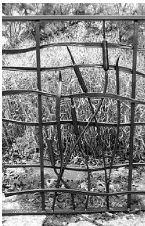
A three-step process follows the hand-rendered sketch (top) of a forged-steel fence through a construction drawing (middle) to the forged, full-scale sample (bottom); courtesy Lars Stanley, AIA.
