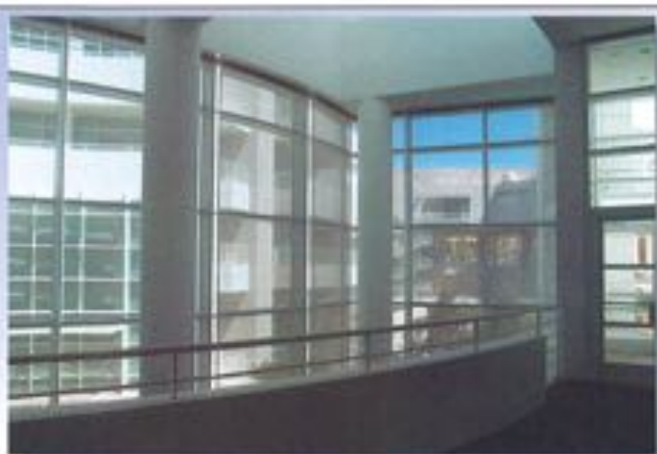
SuperScreen Motorized Shades, Recess Mounted, The Getty Center, Los Angeles, CA
