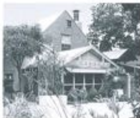
Gardens Addition & Remodel
