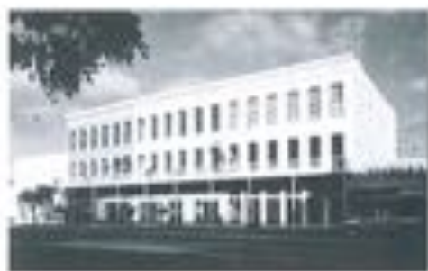
Market Street Lofts
