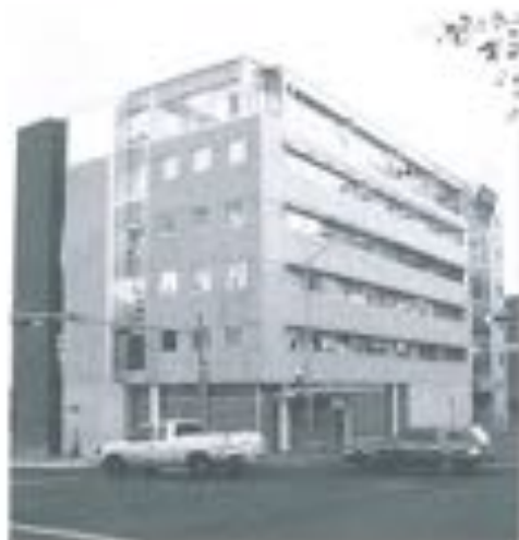
Renovation &amp; Addition: 1011 San Jacinto Office Building
