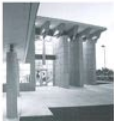
El Paso County Juvenile Courts Facility
