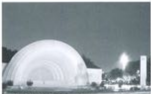
Fair Park Band Shell Renovations
