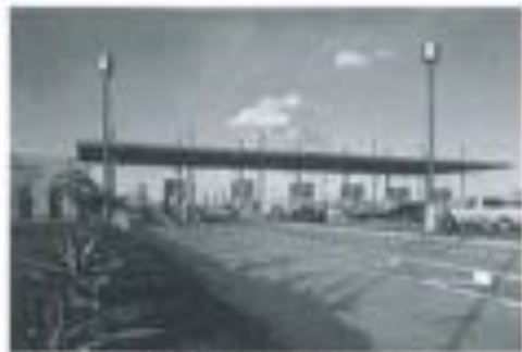
Las Tomates Toll Station & Administration
