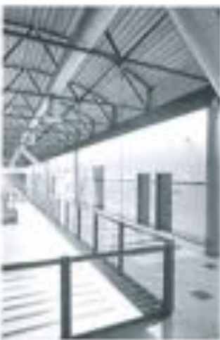
Denton High School Connector Building
