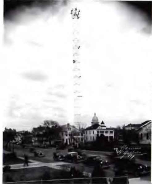
4 historical photo; a worker can be seen mid-way up the tower
