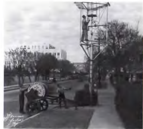
3 historical photo showing workers using the elevator to replace lights
