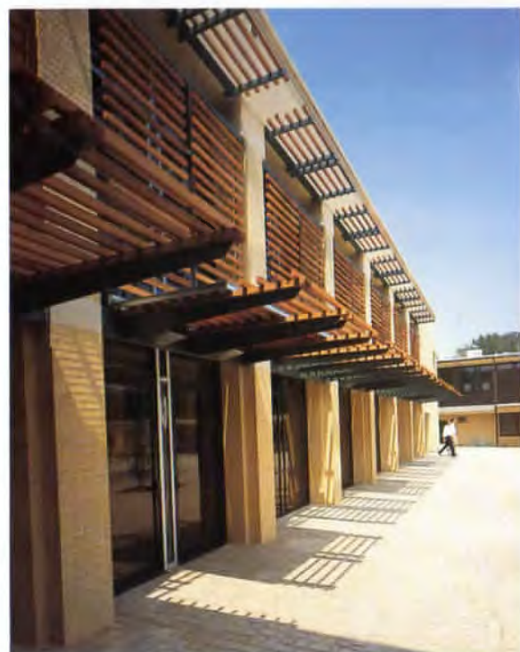
1 St. Pius X Fellowship Hall, looking through the lobby and into the hall from the courtyard
