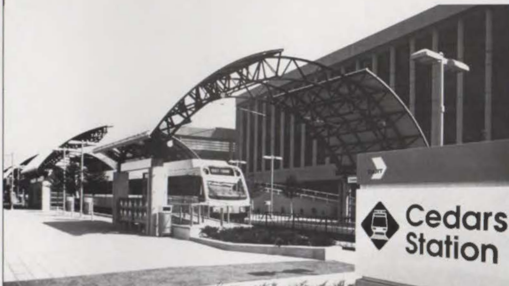
OPPOSING ARCHES FORMED BY BERRIDGE CURVED TEE-PANEL ROOFS ACCOMMODATE HIGH-VOLTAGE LINES FOR ELECTRIC-POWERED D.A.R.T. LIGHT RAIL TRAINS, VIA A CENTER OPENING
