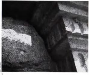
The granite was both cleaned and its joints repointed during the exterior restoration phase.
