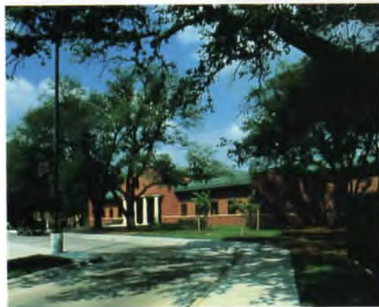
Right and plan: Despite the tight site, a winged arrangement saved trees and enhanced multi-grade activities.
