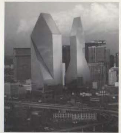
Among an estimated 20 projects in early stages of negotiation in Dallas is the companion to First Interstate Tower (formerly Allied Bank Tower; designed by I.M. Pei and Partners) at Fountain Place. Chubb Realty recently purchased the property.
